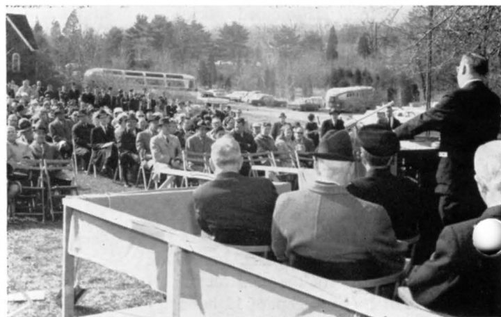
Audience listens as President Thomas L. Morison opens program marking the ground-breaking for 12 new buildings that are expected to be ready for occupancy in the fall of 1968.
